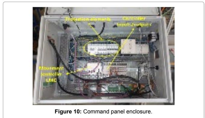
The electrical enclosure includes principally the four speed drives, electrical and human protections equipment (circuit breakers, differential breaker, thermal and magnetic fuse, kill switch, etc...). On the other side, the main task of control panel is to pilot the machine.
