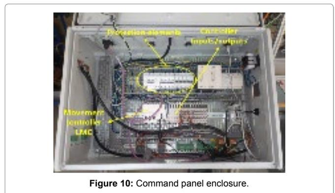
Figure 10: Command panel enclosure.
