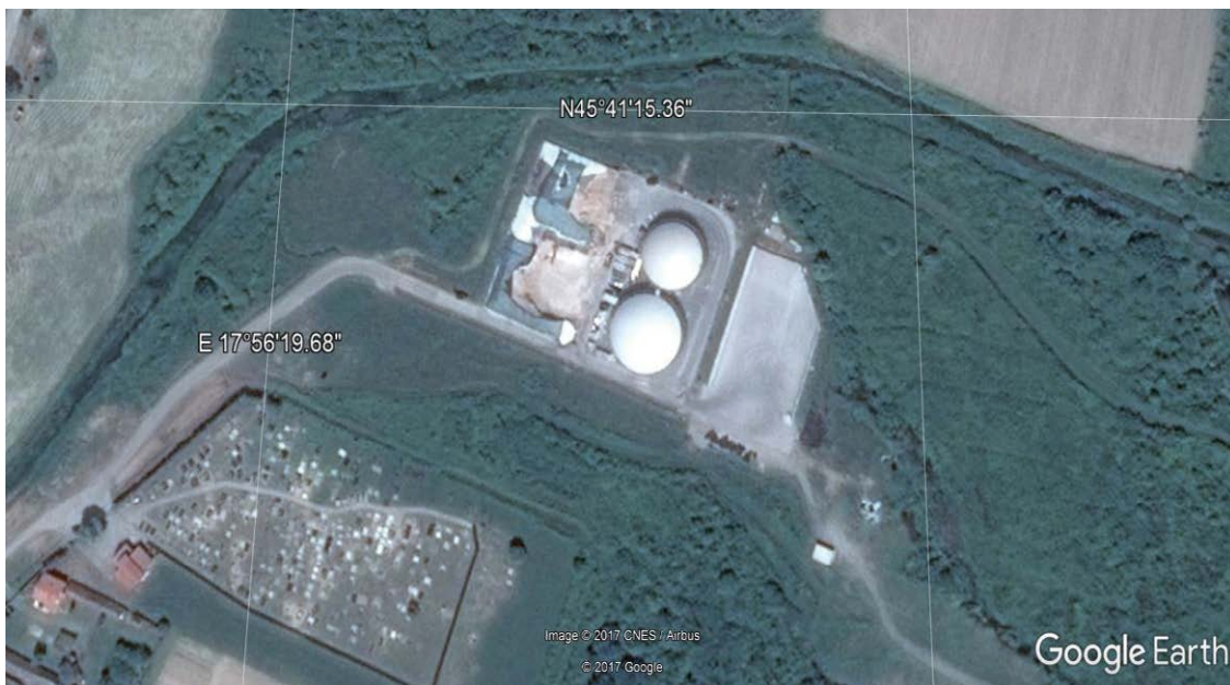
Figure 1: Location of biogas power plant "crnac".
