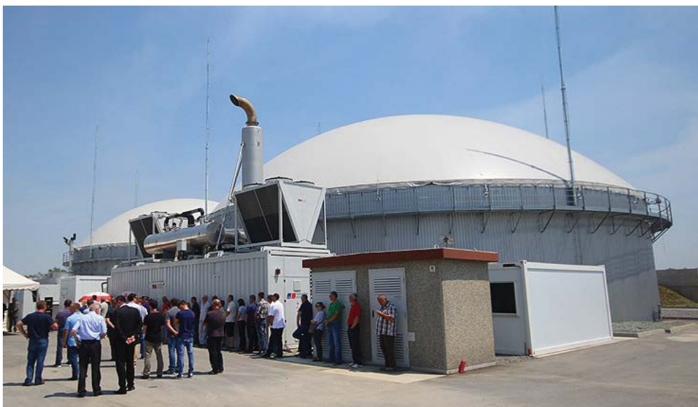
Figure 2: View of the biogas plant.
