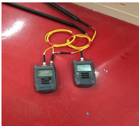
Figure 8: Measurement of power losses.
