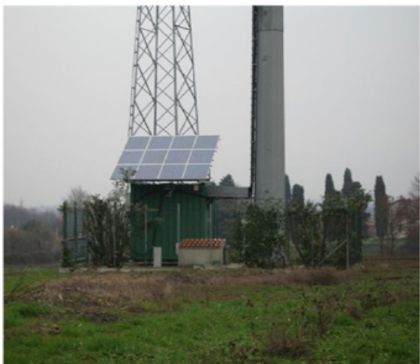
Figure 4: BTS structure design of Photovoltaic (PV) applications.
