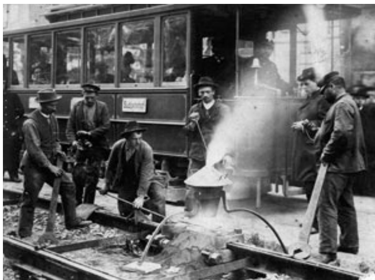
Figure 15: Welding rails by the Thermit process.
