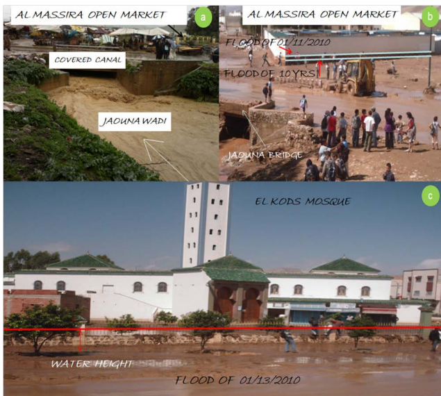
Figure 2: Properties placed into floodable area of the Jaouna Wadi. (a) Al Massira open market in flood-prone area. (b) Al Massira Market after the flood of 13/01/2010. (c) El Kods Mosque after the flood of 13/01/2010.
