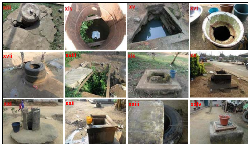
Figure 12b: Dug wells in Kumba. Most fall short of the [24] specifications for the completion and protection of hand-dug wells; xiii) broken apron: unsafe, facilitated direct pollution, in need of rehabilitation, xiv) grass growing in well, xv) no cover, no collar, no concrete apron, really shallow and open: possible breeding ground for mosquitoes, very susceptible to direct pollution, xvi) inappropriate cover, no apron, xvii) no cover, used car tire collar, xviii) inappropriate cover, no collar, no apron, grass growing on well with resident bats, xix) no cover, broken collar, xx) no cover, broken collar, xxi) no cover, broken collar, xxii) no cover, xxiii) used-car tire collar, inappropriate cover, no apron, xxiv) no apron.
