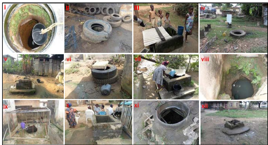
Figure 12a: Dug wells in Kumba. Most fall short of the [24] specifications for the completion and protection of dug well; i) no cover, growing grass visible, ii) no concrete apron, used car tire as collar, stores water which is potential breeding ground for mosquitoes, no cover, vulcanizing activities too close to well is a potential source of pollution, iii) no gate, inappropriate cover, danger to children (cases have been reported of children drowning in wells in Kumba, iv) no concrete apron, used car tire collar, no cover, v) no cover, broken collar, too close to pit latrine, vi) inappropriate cover, used car tire collar, poor care of well rope and bucket, vii) inappropriate cover, viii) no cover, no collar, no concrete apron, really shallow and open: possible breeding ground for mosquitoes, very susceptible to direct pollution, ix) broken collar, no cover, x) no cover, xi) no cover, broken apron, badly in need of rehabilitation, xii) no cover, broken collar and apron.
