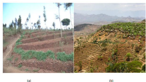
Figure 3: The Konso dry stone-walled agricultural terraces. (a) Near view of the bench terraces; (b) Far snapshot view of the terraces.
